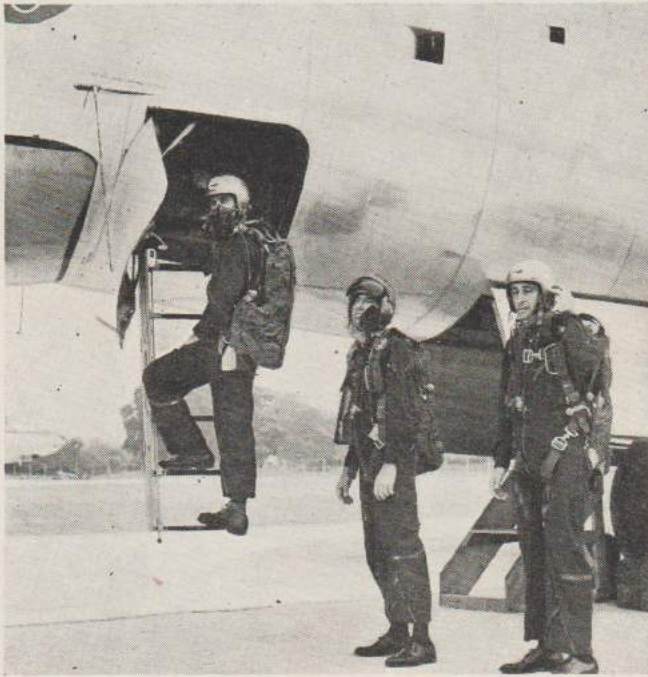
Left, Major L. E. Gunter, and Capt. R. R. Barto and A. T. Brent, of the 369th Sqn., enter their B-47. Note their helmets, visors and extra-bulky parachute packs. Right, this view of the B-47 shows the marked ground anhedral of the wing. The bulge beneath the cockpit houses radar gear, while in the extreme nose is an optical bomb sight. Below, pilot and co-pilot in their long cockpit, with the radio compass aerial in between.
