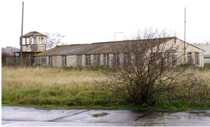
Fig 1 Typical Maycrete building
